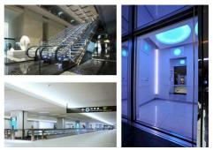
1. Reduced speed control: The escalator shall change to a slower speed when no activity has been detected for a period of a maximum of three (3) minutes. Detection shall be by photocell activation at the top and bottom landing areas.
